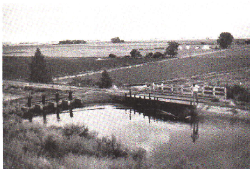
WALDVOGEL CANAL HEADWORKS AND MORA CANAL DROP INLET
