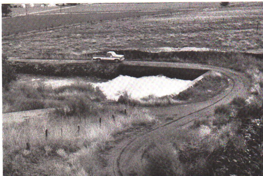
MORA CANAL DROP STILLING BASIN
