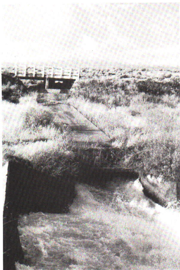
MORA CANAL DROP CHUTE AND STILLING BASIN
