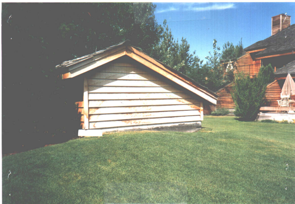
Pumphouse for well no. 1 Looking south- west
