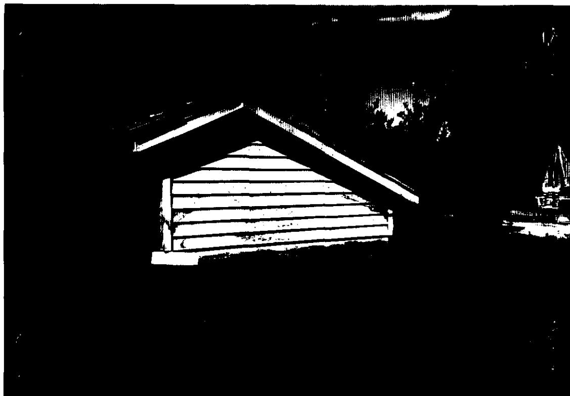
Pumphouse for well no. 1 looking south- west
