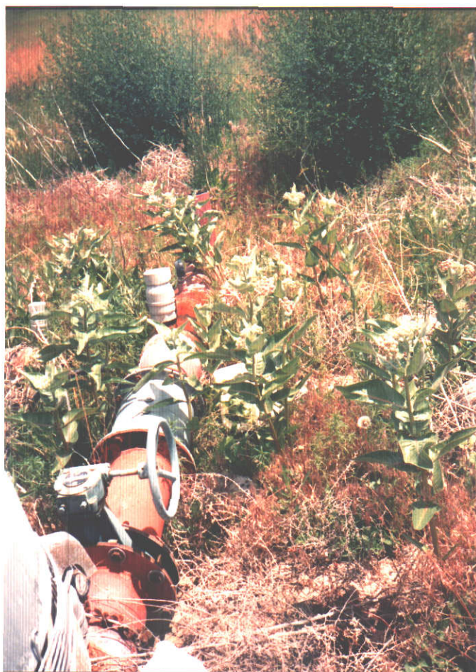
#2. Discharge line and site where pipe from 2nd well connects to the discharge from this well. Discharge line from this location goes under- ground but resurfaces about 600' South.
