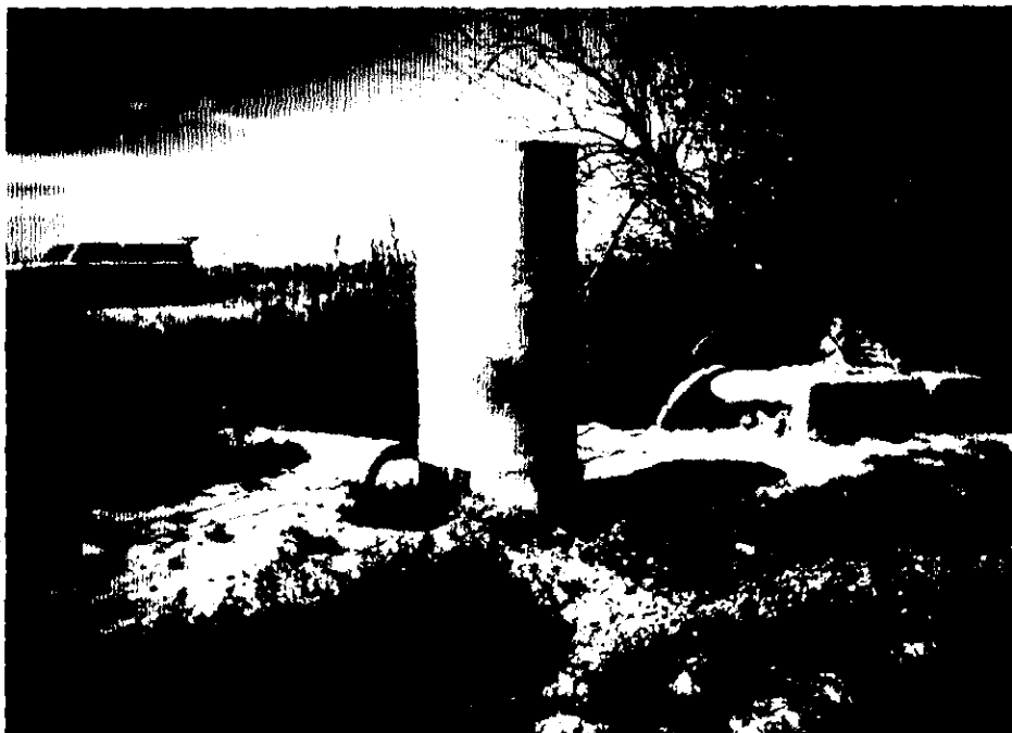
#2 Collection tower that receives water from a buried 12" pipe prior to delivery under Hwy 20-26 to the P/D. This tower is located North of the highway.
