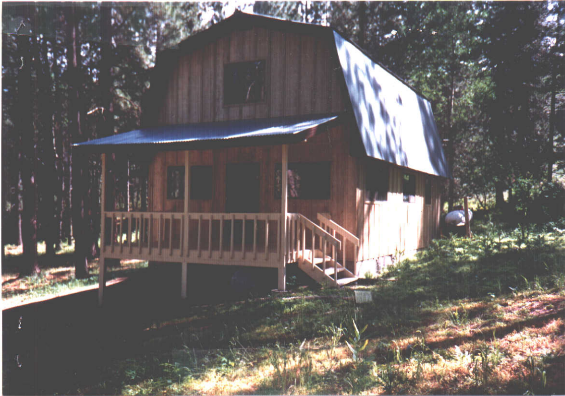
P. U cabin Looking East
