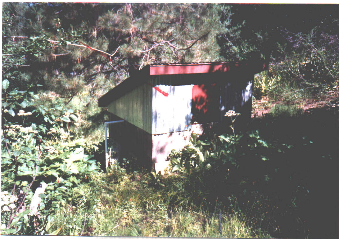
Storage tank with protective structure Looking NNE
