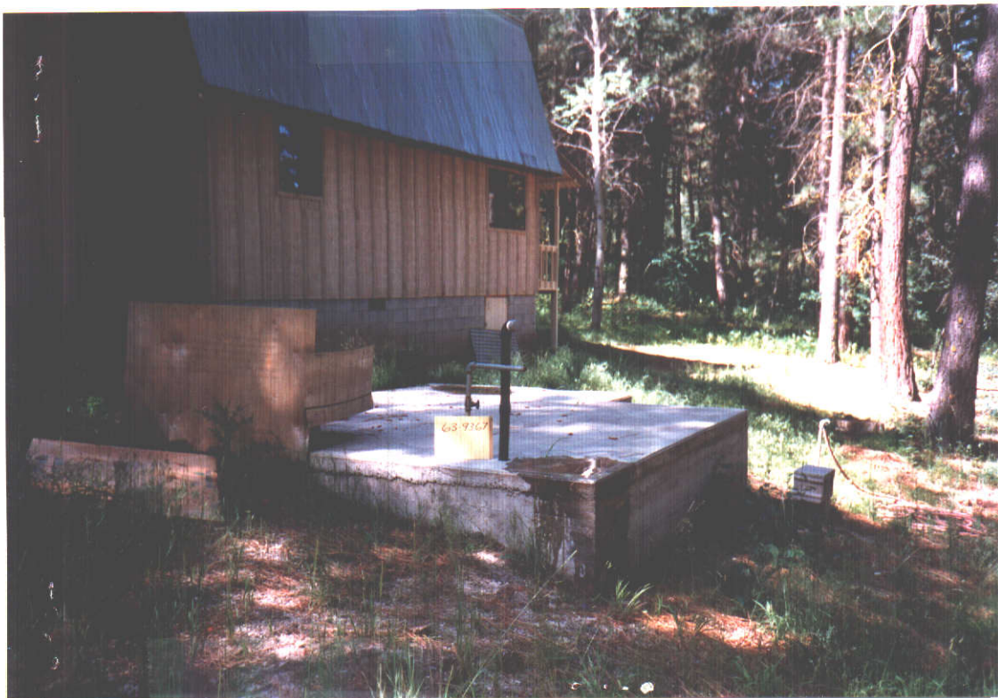
5 gallon bucket filled from the pipe in in the concrete pad Looking West
