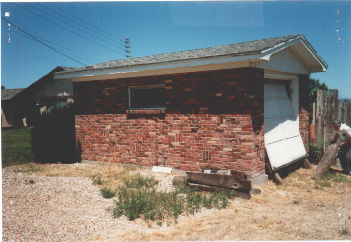
P.D. Well #3 Brick and wood pumphouse 12'11" x 17'8" Looking Northwest
