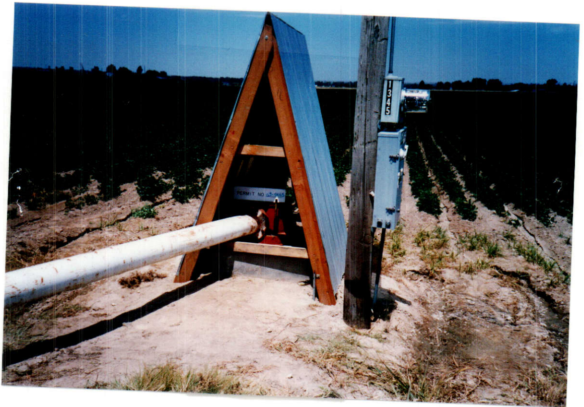
Point of Diversion Looking Northward Place of Use in Background
