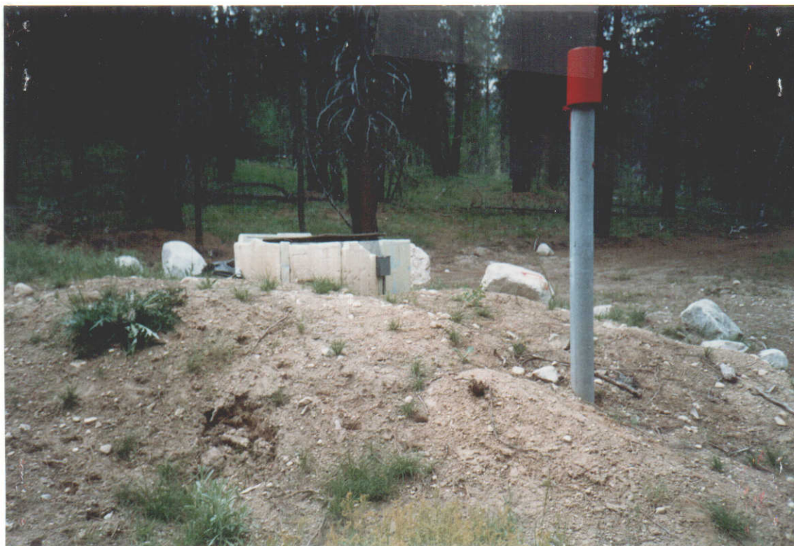
Top of 5000 gallon under- ground storage tank.
