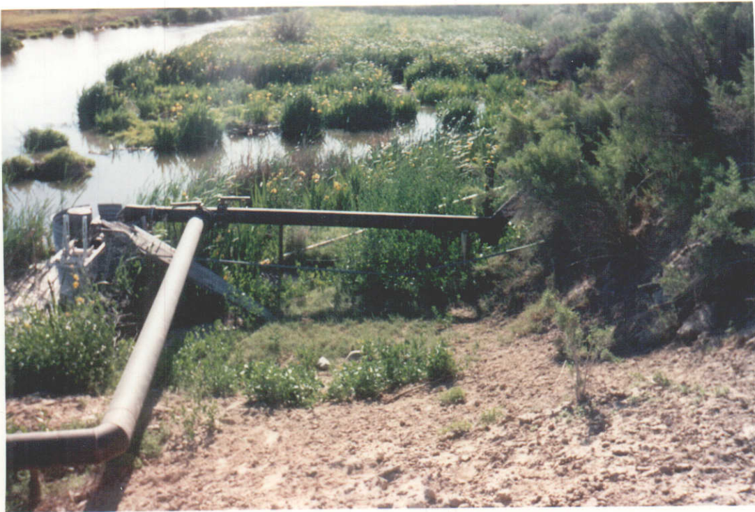
#2 Point of Diversion and discharge pipes.
