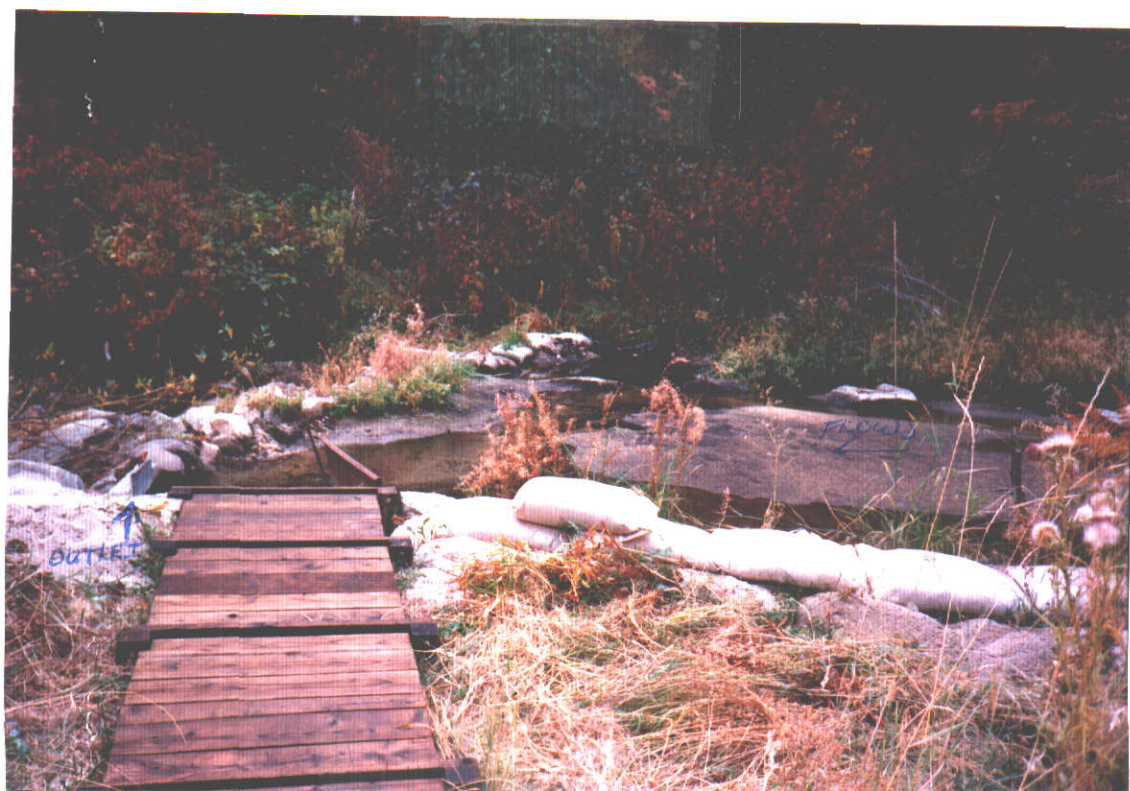
PICTURE No. 2 DIVERSION DAM AT POINT OF DIVERSION WITH OUTLET TO THE LEFT OF FLUME. PICTURE TAKEN FACING SOUTH.
