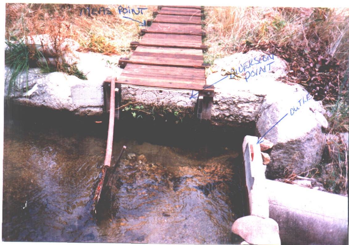
PICTURE No. 1 POINT OF DIVERSION FROM MACK'S CREEK. FLUME IS UNDER WOODEN WALKWAY. MEASURING POINT WAS ACCESSED BY LIFTING UP BOARDS IN WALKWAY. PICTURE TAKEN FACING NORTH.
