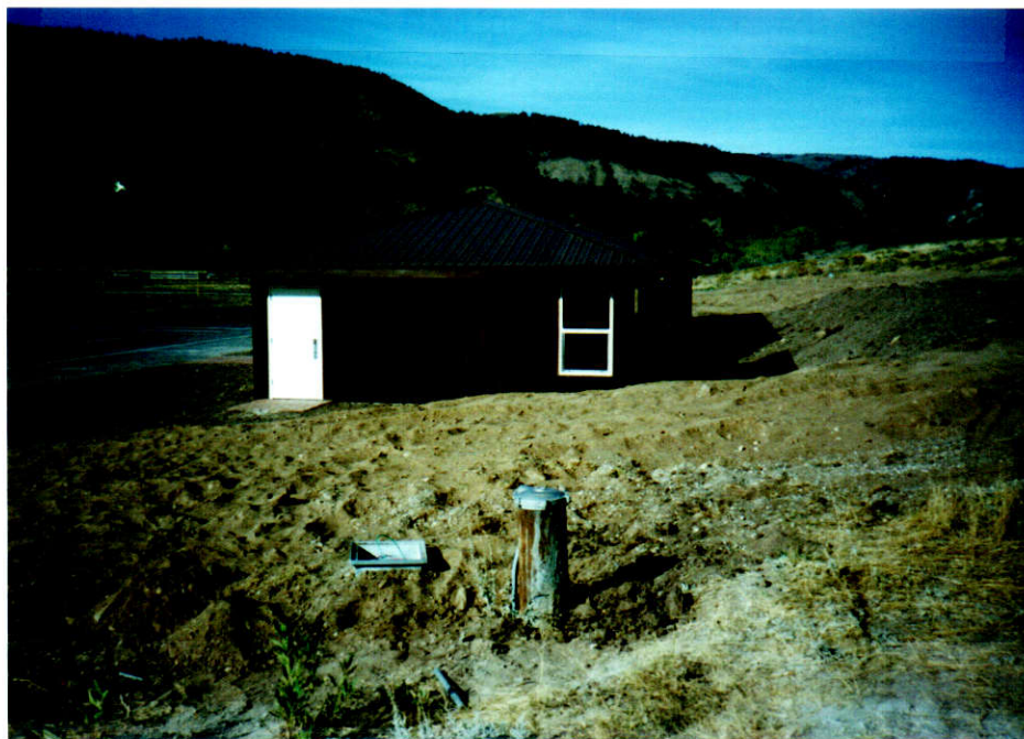
Fig. 1 - Point of diversion showing shower buildings.
