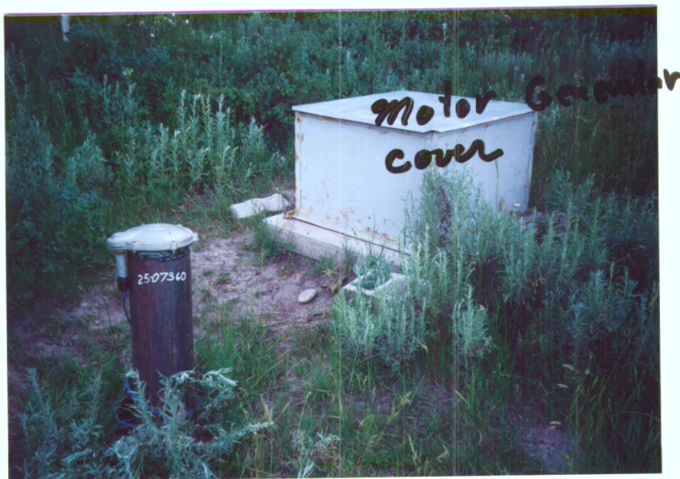
Well and generator Motor Cover looking West.
