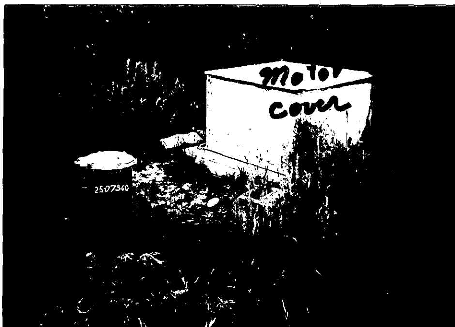
Well and generator Motor Cover looking West.
