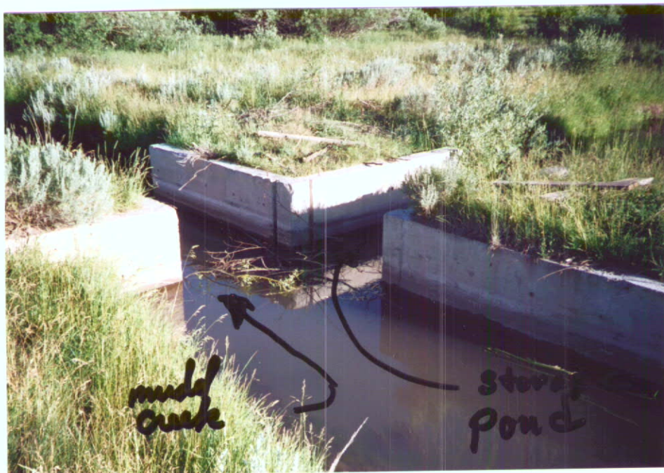
Looking South at inlet to pond and mud Creek
