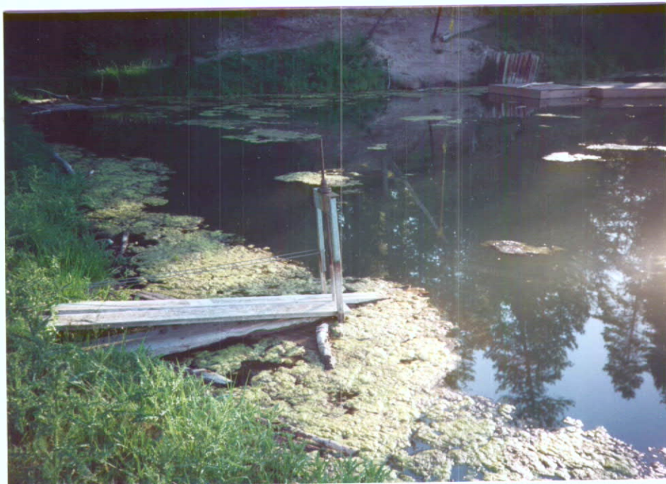
pond outlet looking South West.
