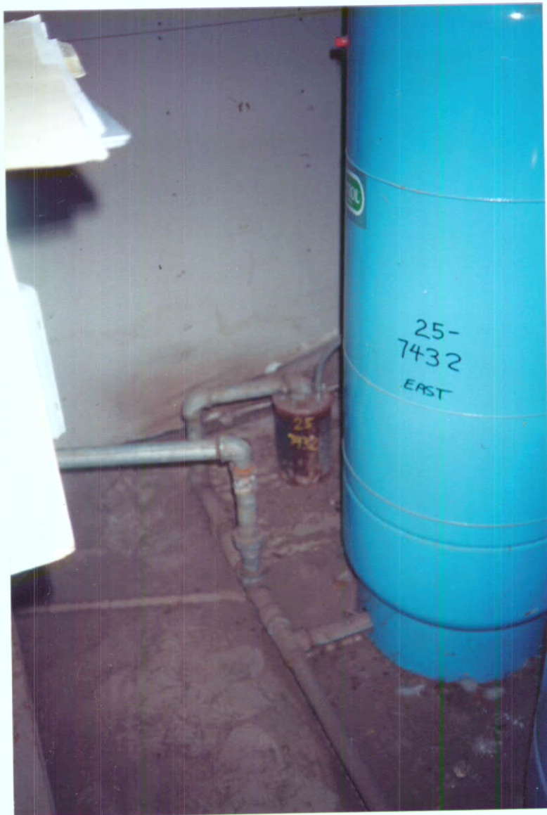
EAST WELL 6/76 drilled
