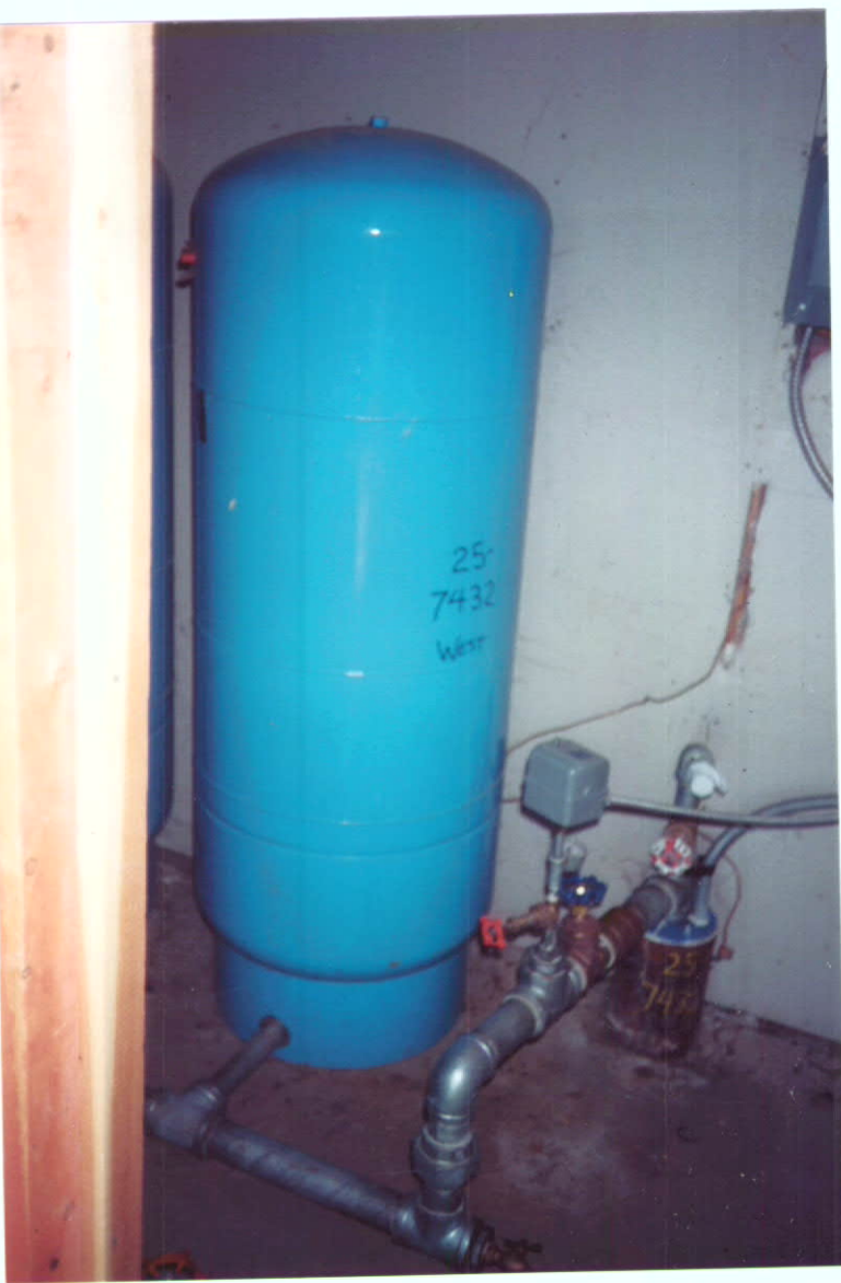
WEST WELL 5/76 drilled
