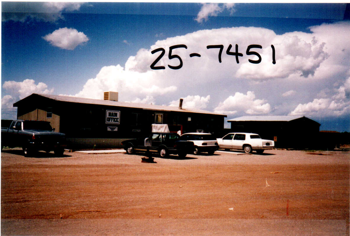
OFFICE BUILDING - PLACE OF USE
