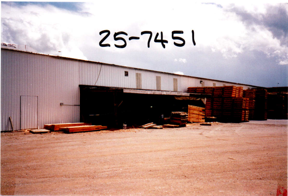
Roller Plant - View 2
