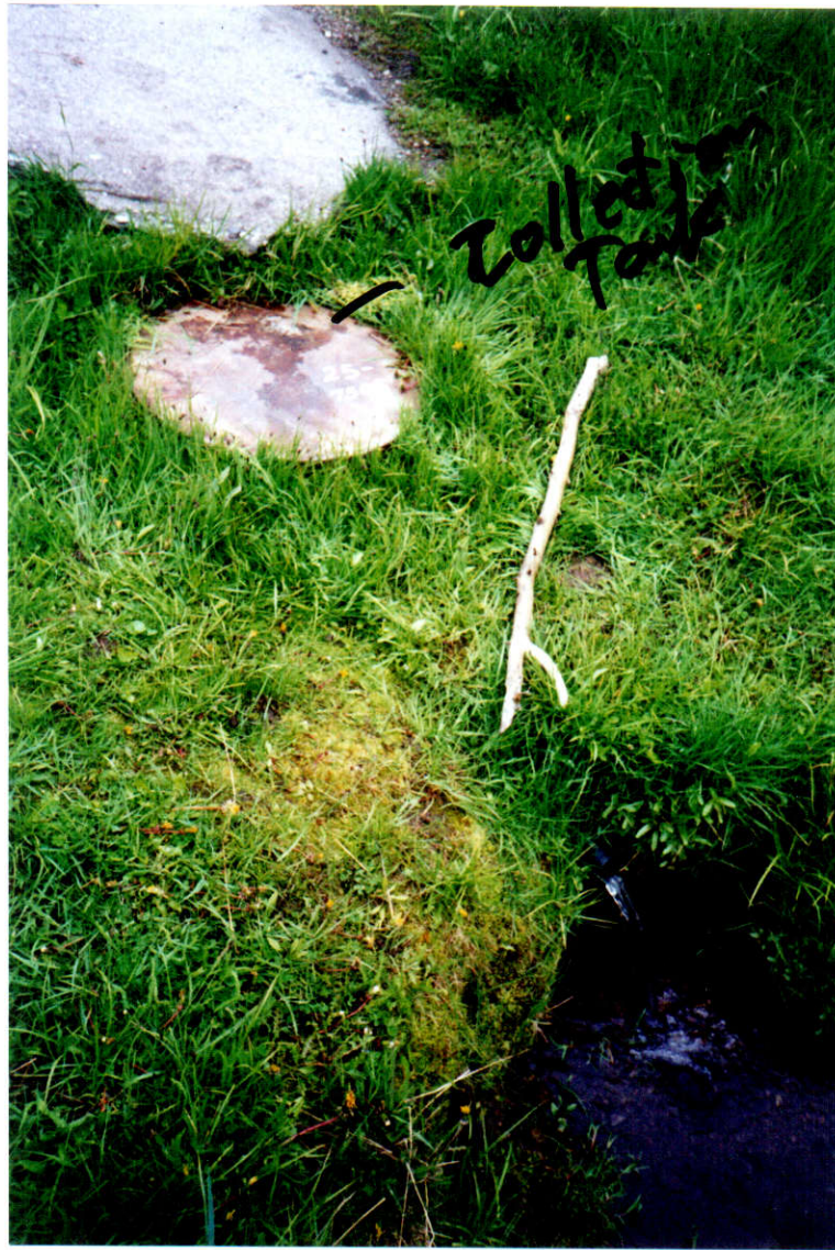
Spring outlet with collection Drum and concrete cap in top of photo - looking South
