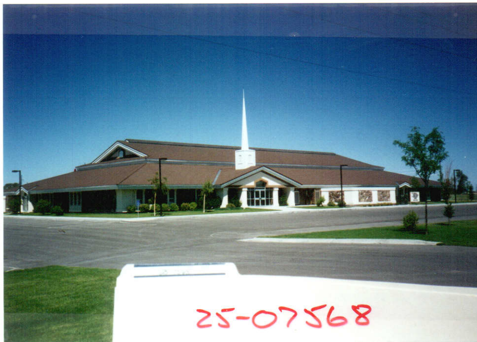
Fig. 2 - Church building and lawn area at place of use.
