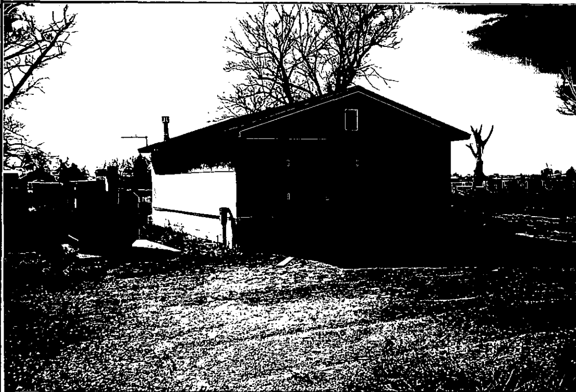
WELL HOUSE LOOKING SOUTH WEST
