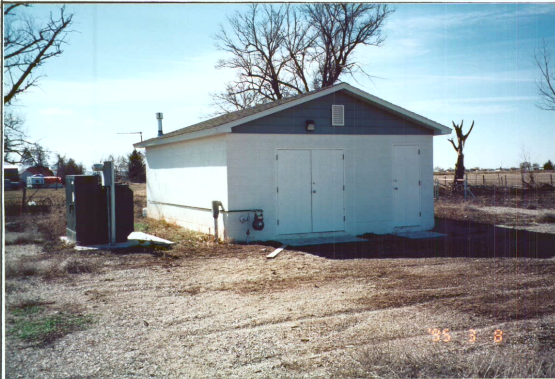
WELL HOUSE LOOKING SOUTH WEST
