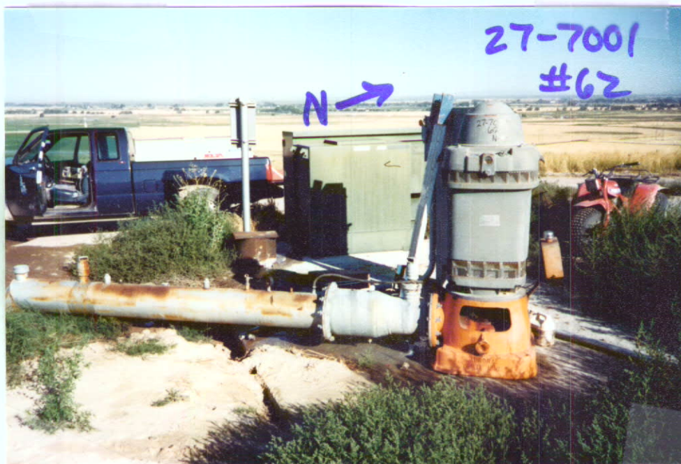
Point of Diversion #62
