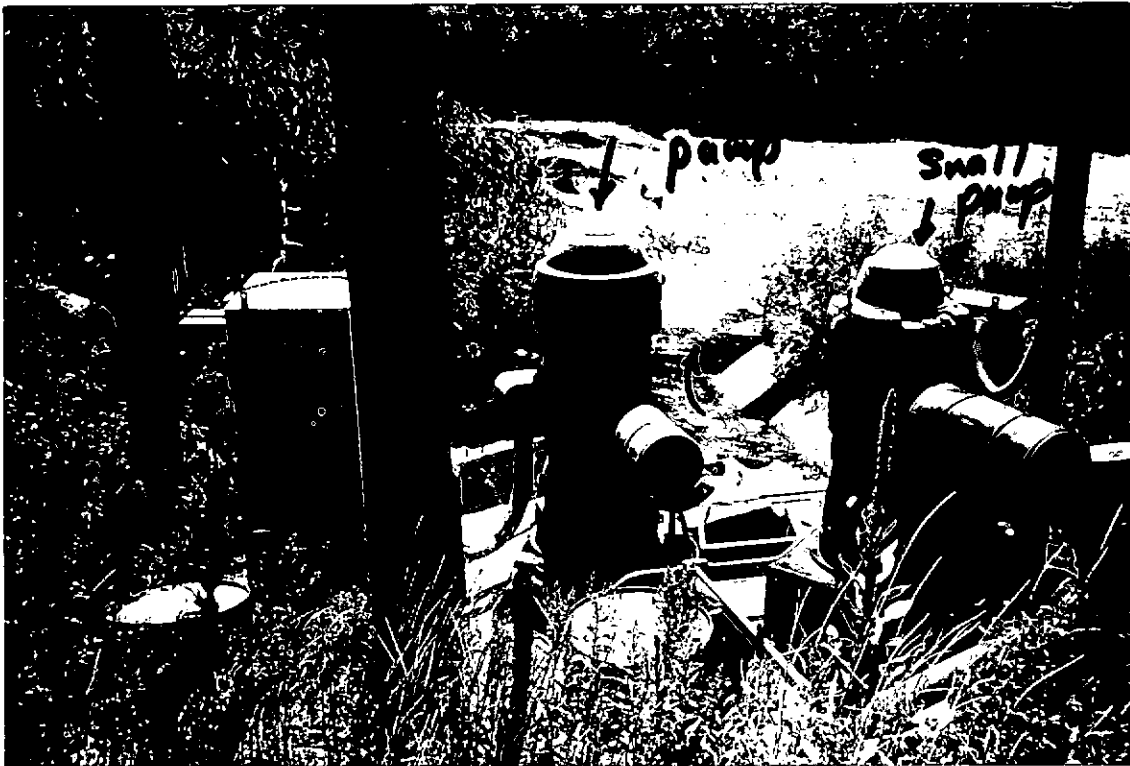
looking South at large Pump (left) and Small pump (Right). channel returning excess water back to river. Diversion Pipe shown on left
