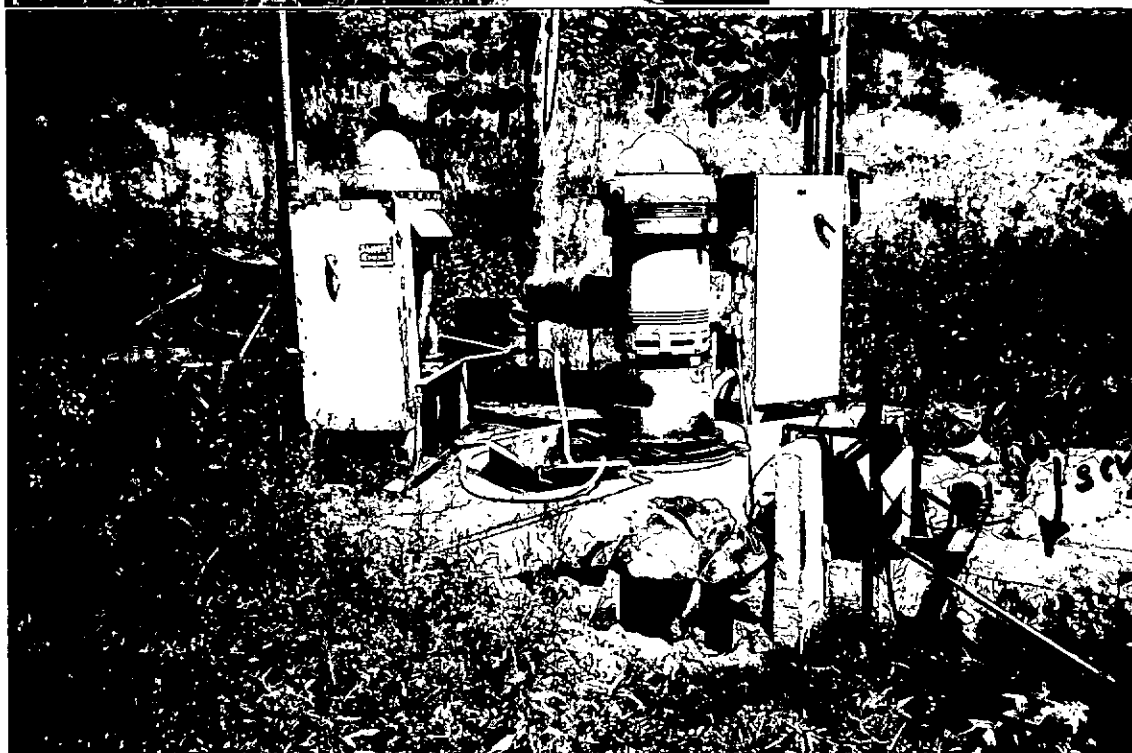
looking North East at pump arrangement,
