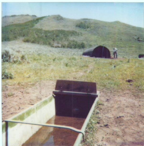
BADGER KNOLL TROUGH & STORAGE TANK
