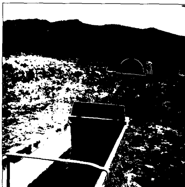
BADGER KNOLL TROUGH & STORAGE TANK
