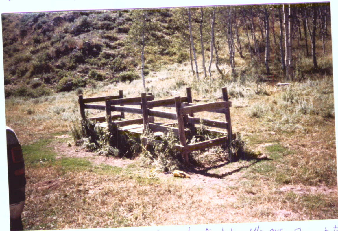
Spring Area - Looking North East. Spring was developed with gravel + 4" perf. pipe that drains into 1 1/2" pvc pipe
