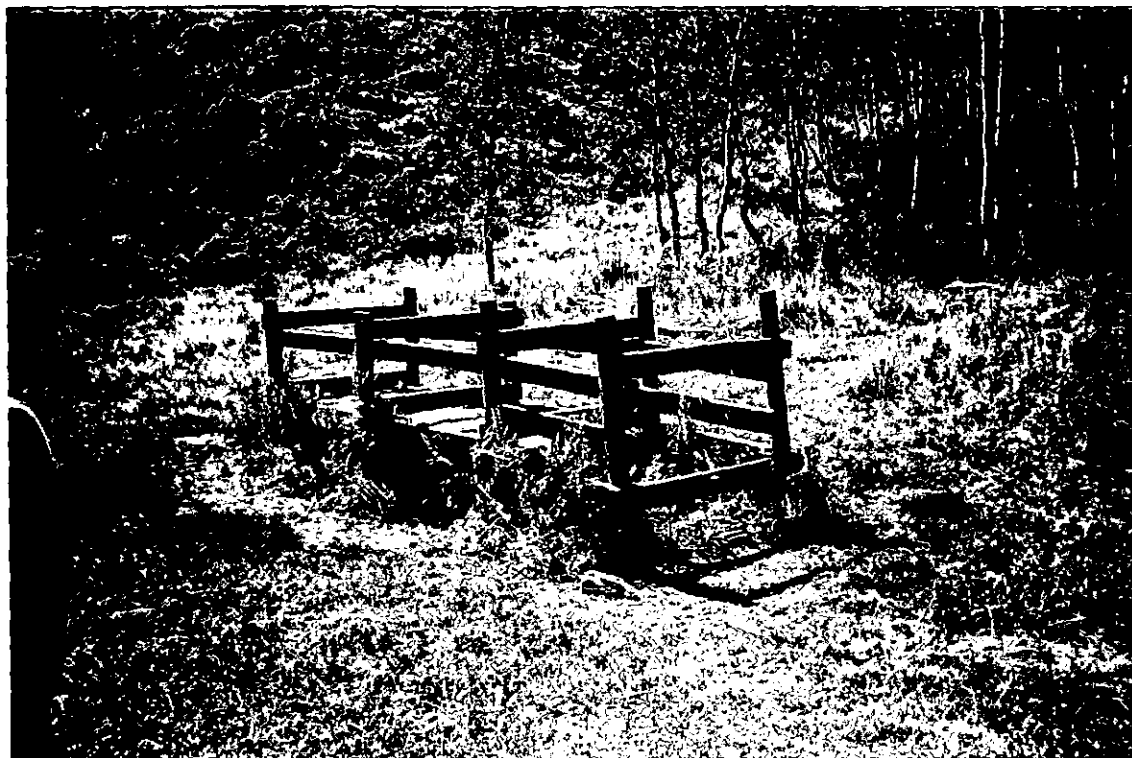
Trough Upper looking South West. Feed by 1 1/2 pvc Pipe and has a flat to Control Water level. Permit # 27-7370
