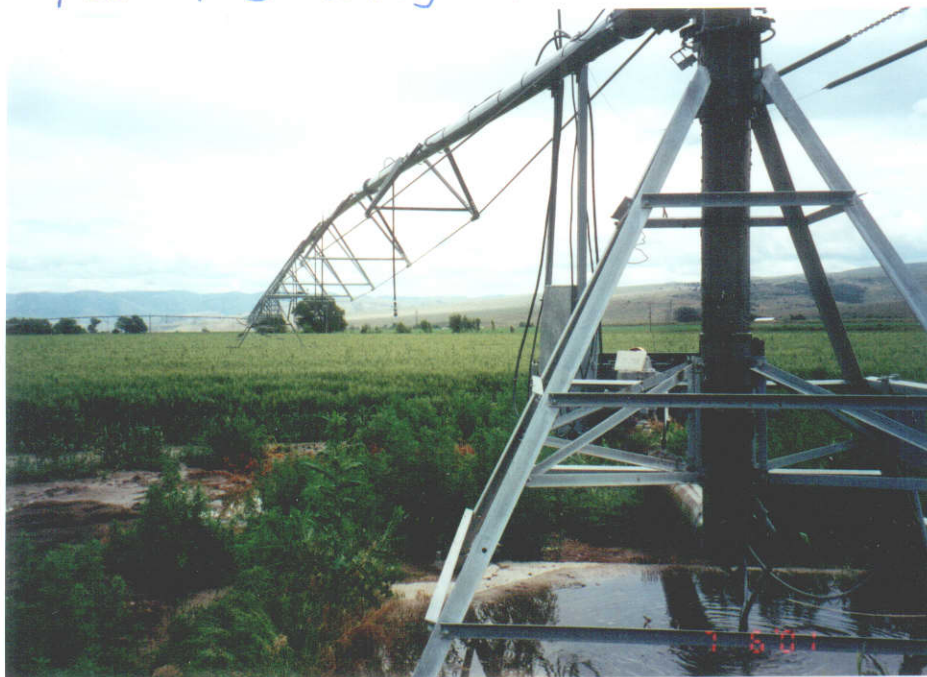
POU + POD looking east
