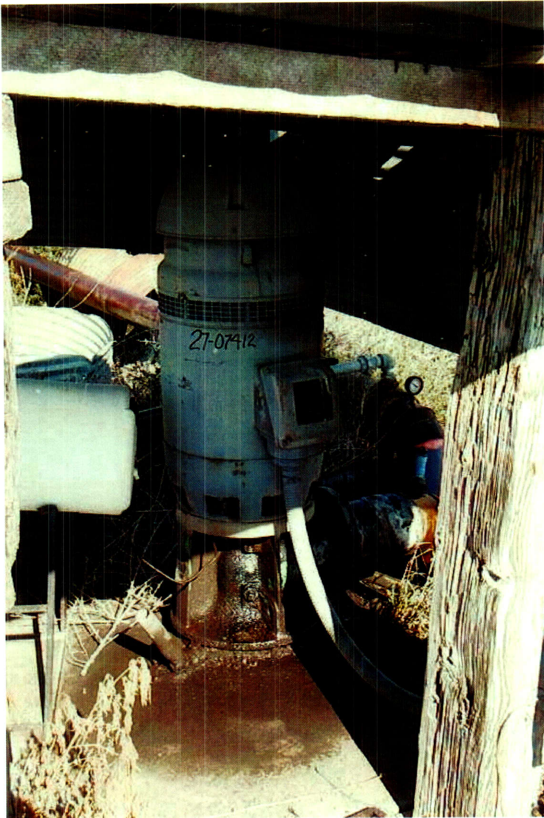
Point of Diversion
