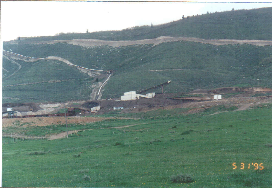
DISTANCE VIEW OF WASH PLANT PLACE OF USE
