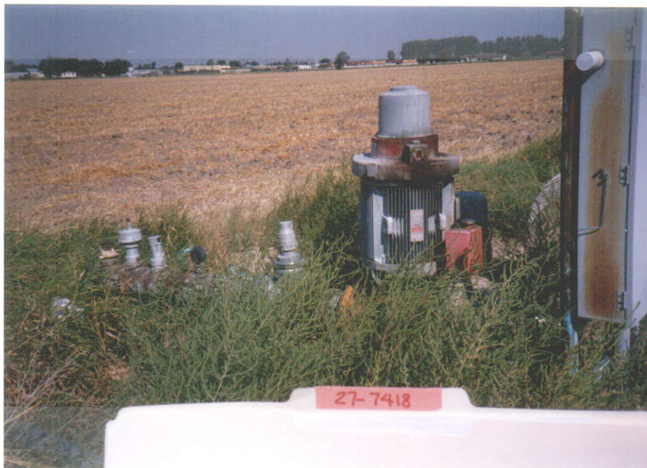
Fig. 2 - Point of diversion looking northwest over place of use.
