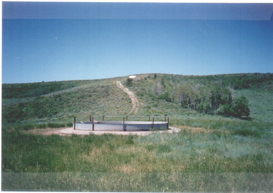
STOCK WATER TROUGH, LOOKING BACK AT TANK AND POINT OF DIVERSION.
