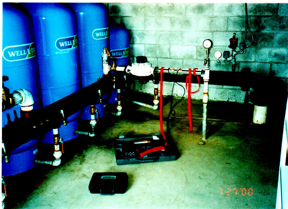
1 hp pump measurement
