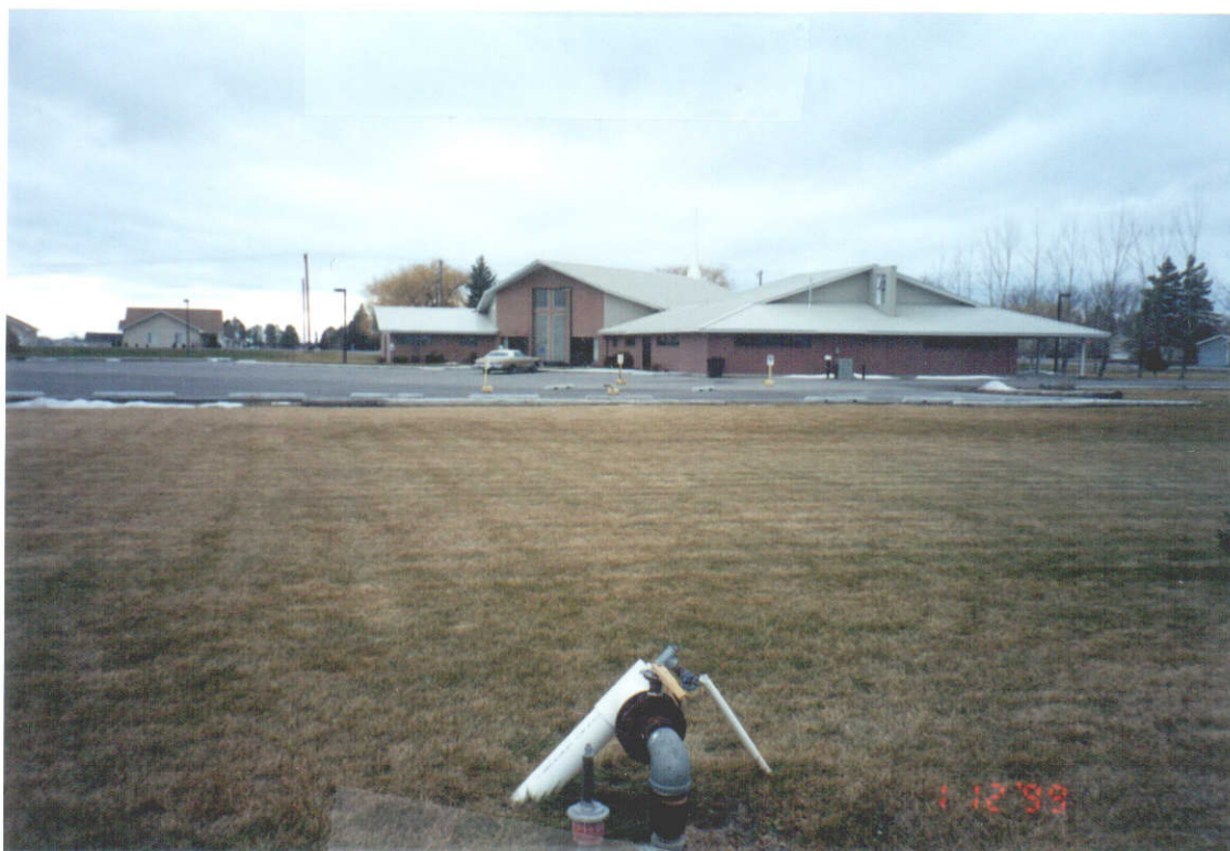
Plate 3 - Place of use looking NW towards church building.
