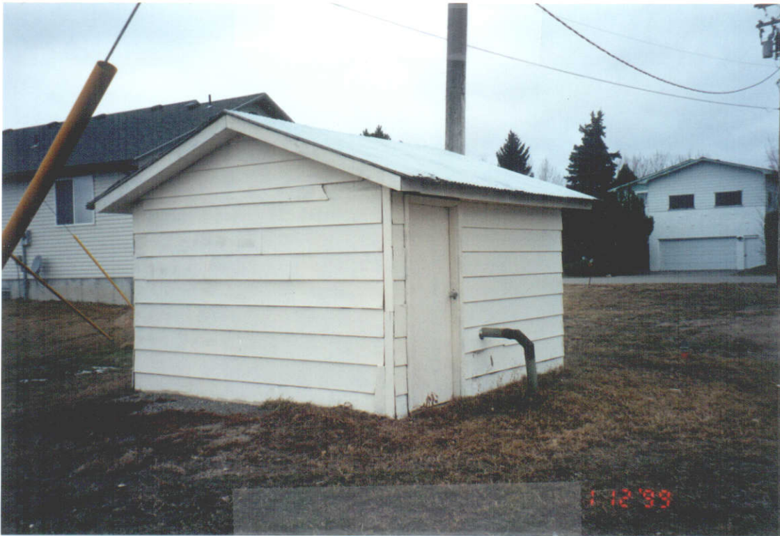
Plate 2 - Pumphouse at point of diversion.
