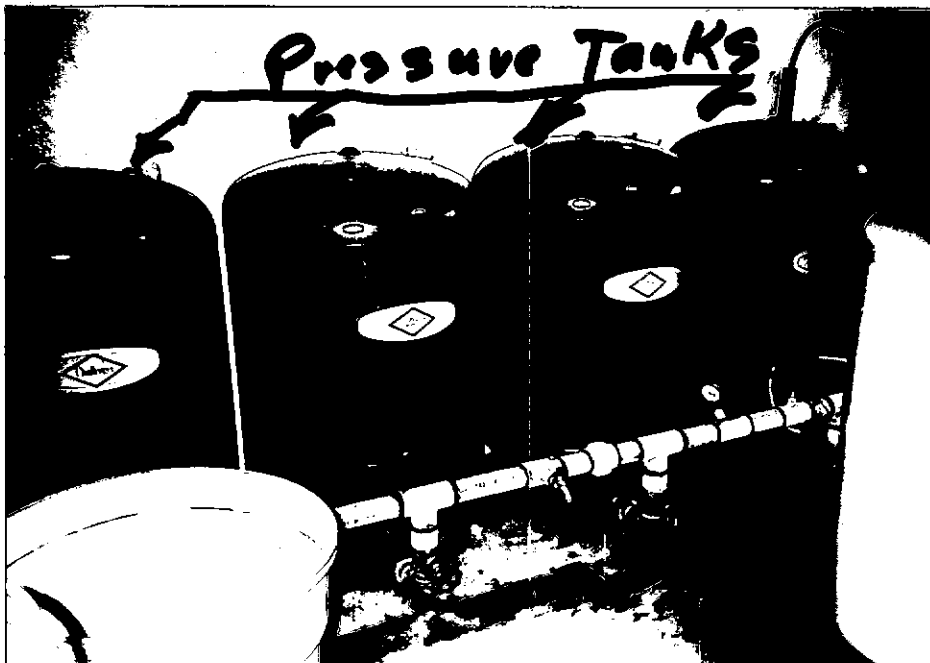
looking east at Pressure tank (4)
