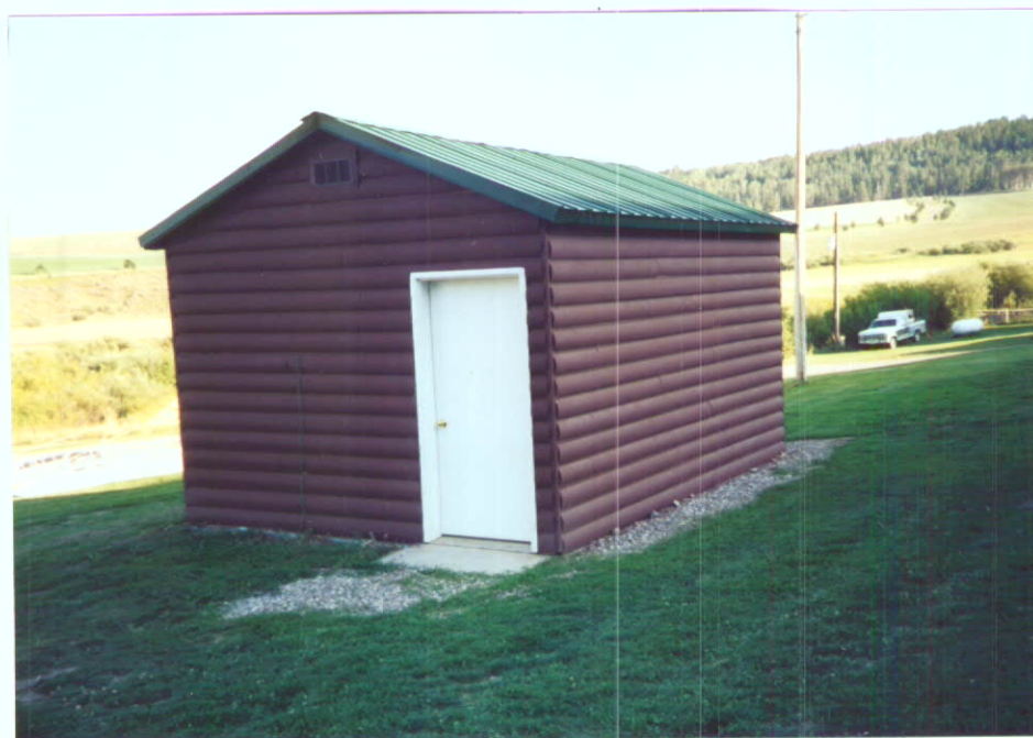
Pump house looking South East.
