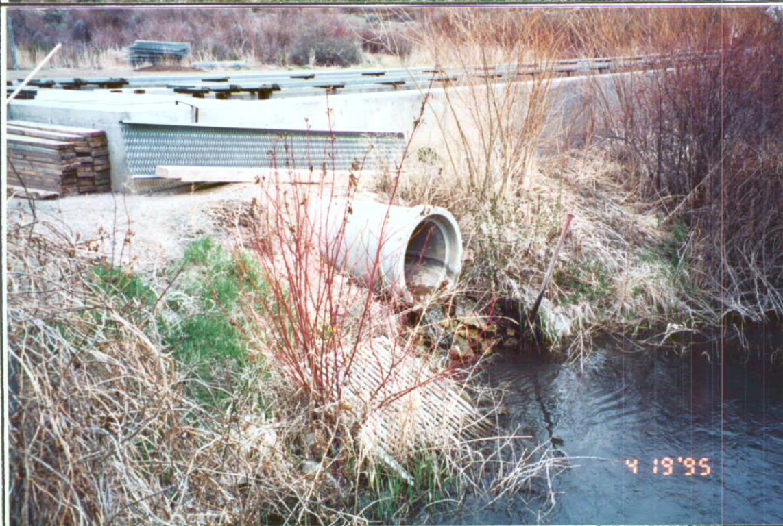
VIEW OF 3RD BYPASS DISCHARGE FROM LAST HOLDING PONDS. BACK TO RIVER.
