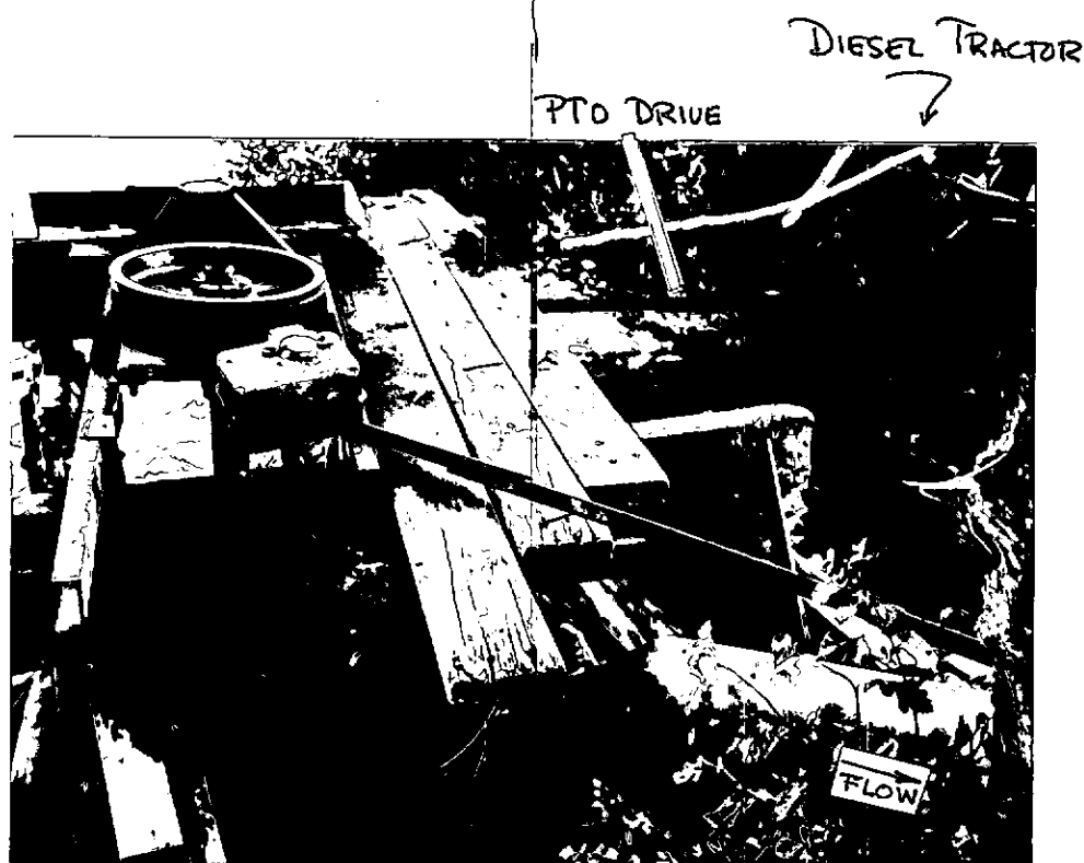
PHOTO # 6 DIVERSION SYSTEM MAINLINE TO OPEN DISCHARGE
