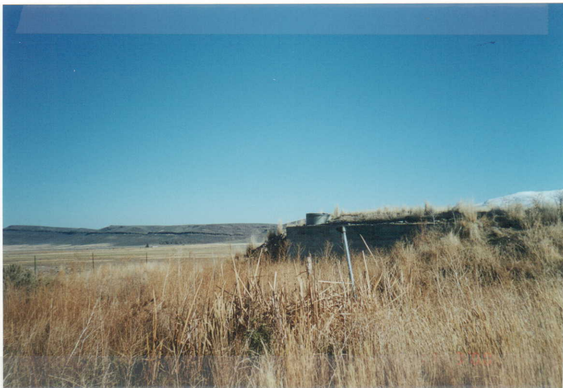
Overflow Pipe On West Side of Storage Tank
