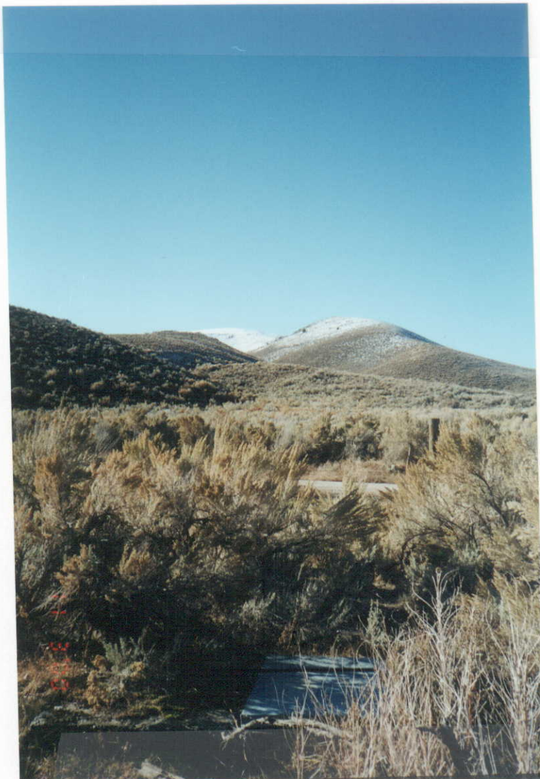
NOWC North Diversion Looking West Across Birch Cr. Road
