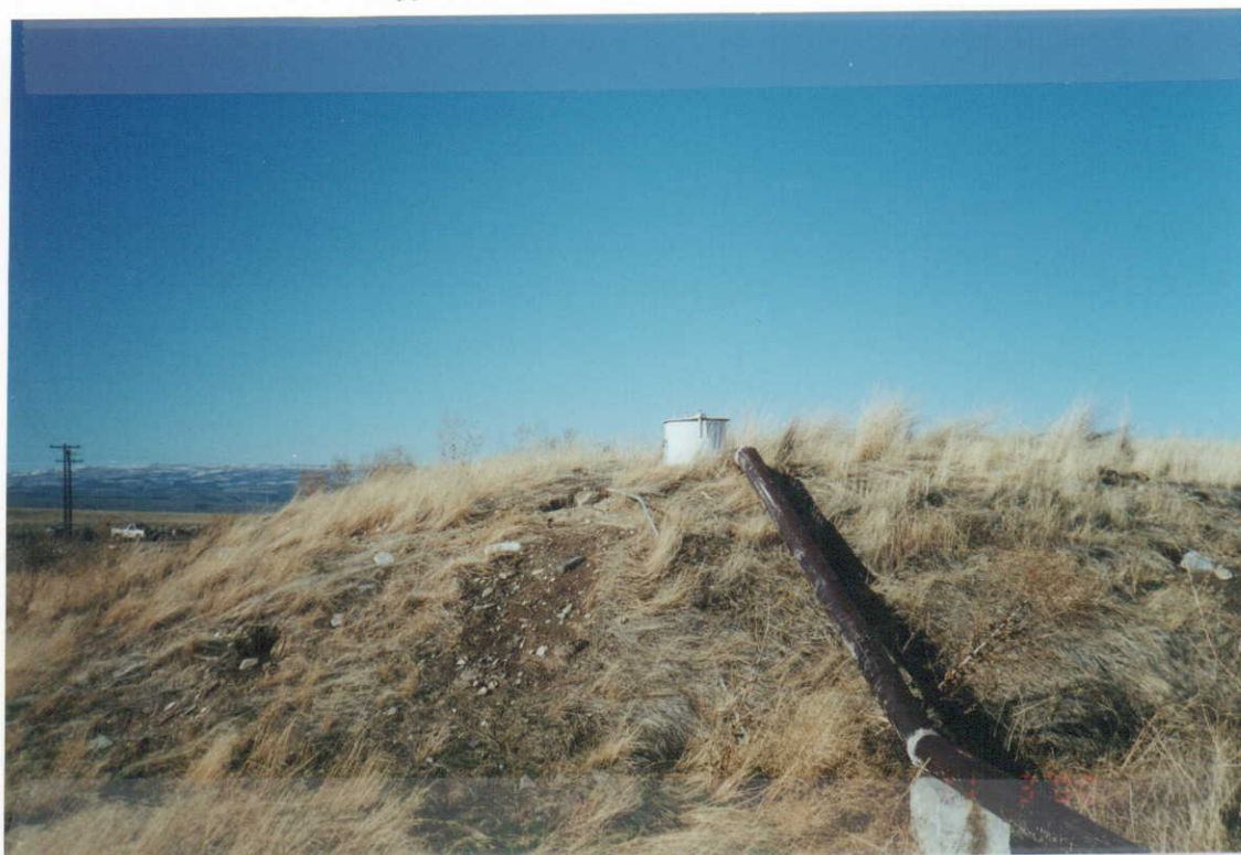
Pipe way Running West From Well To Storage Tank
