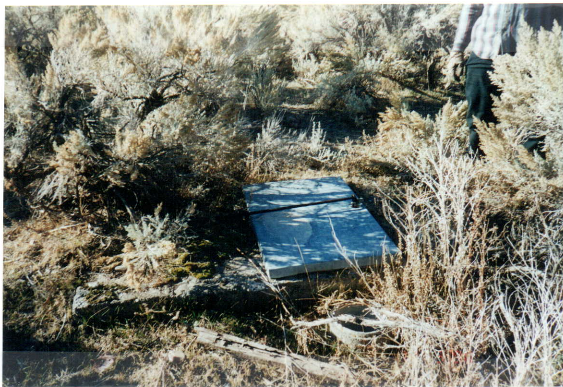
NOWC Lower (North) Diversion
