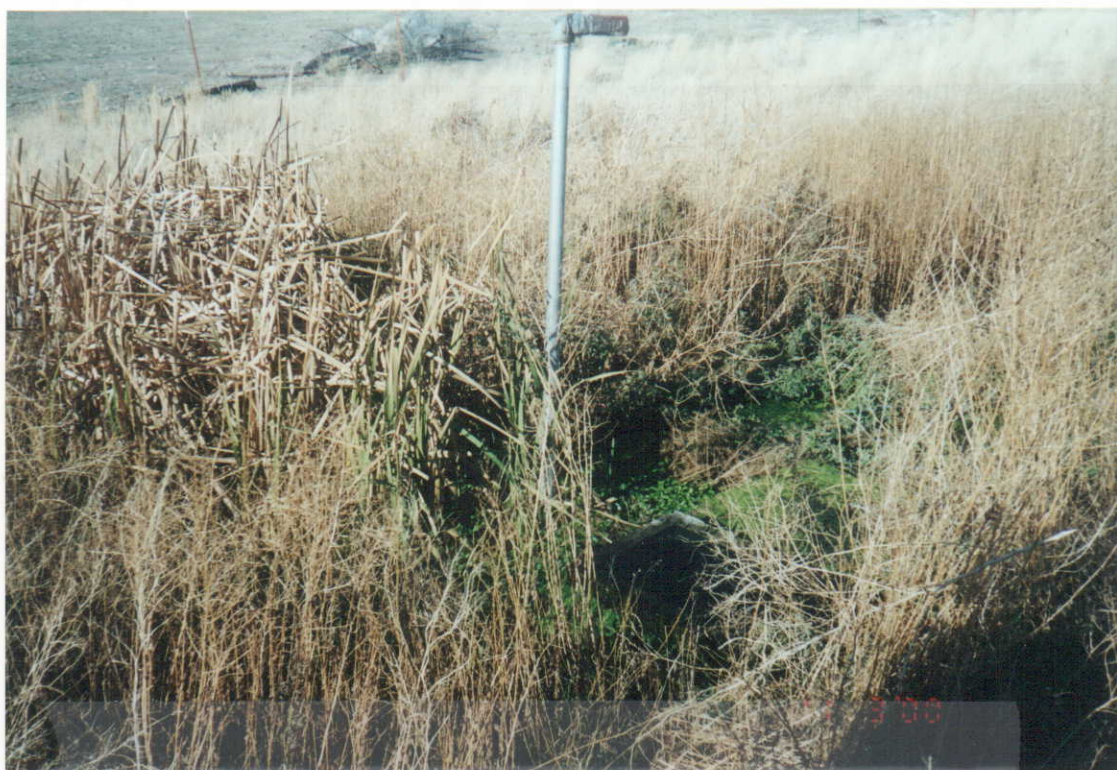
Closeup View (Note Seepage Around Pipe)
