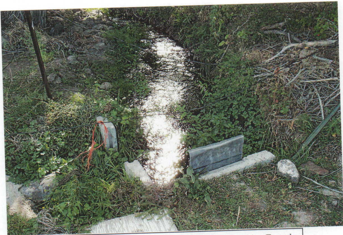
Diversion From Main Ditch To Side Ditch Looking Easterly (Metal Gate Controls Side Ditch) By J E Stanton 9-9-03 App. 47-17100
