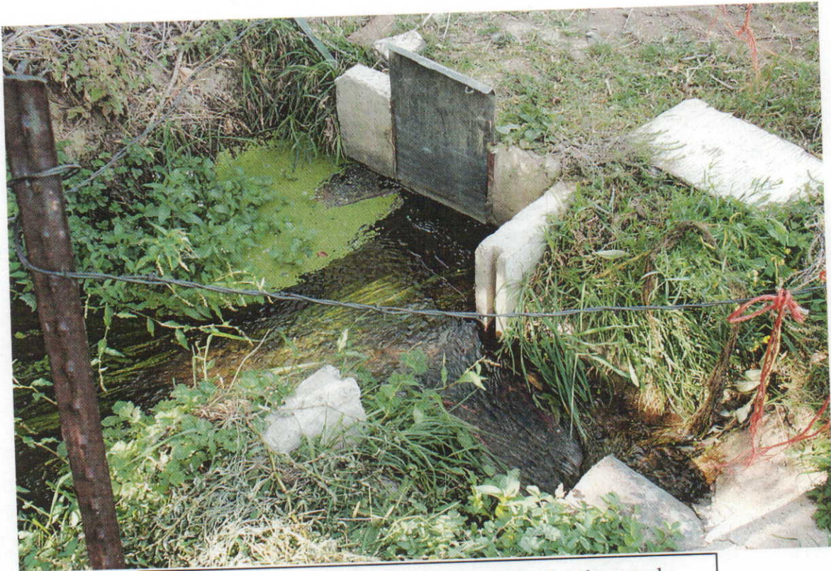
Controlling Works To Side Ditch Looking Southwesterly By J E Stanton 9-9-03 App. 47-17100
