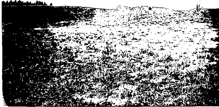
11. The west abutment of the dam connects to this ridge on the far side at approximately the marked place. Note the spring and its drainage path in the foreground. This spring flows from the same formation the dam ties to.
