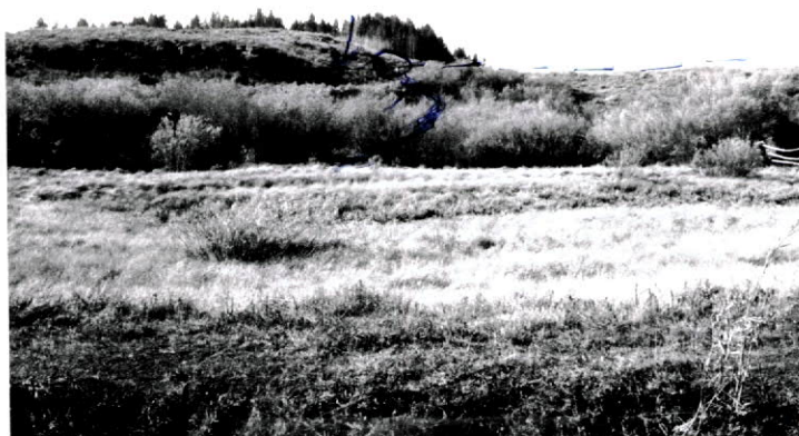
8. Closer view of the area covered by photo 7. The highest evidence of water is circled and flow path roughly sketched in. Note that the highest part of the wet area is well above the dam crest.
