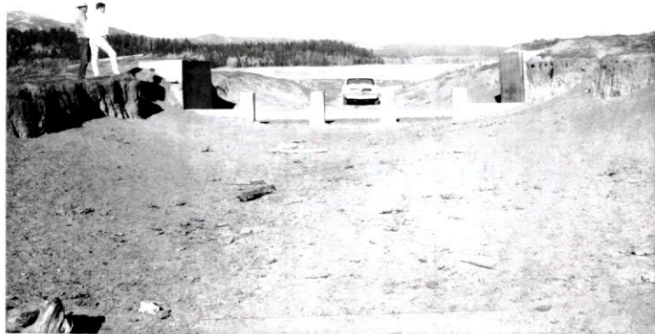
6. New spillway from upstream. Note the gradual slope of the channel. Riprap hasn't been needed since the structure was built in 1963 but will be placed if needed.
