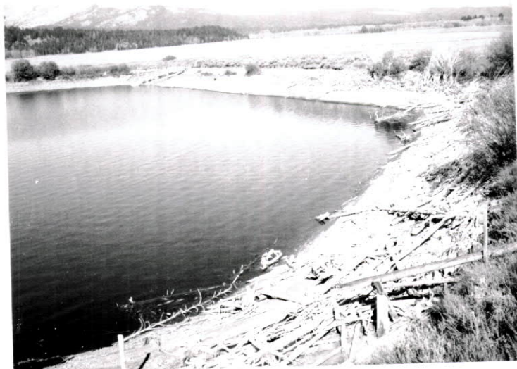
3. Overall view of dam showing riprap, outlet works, and debris.
