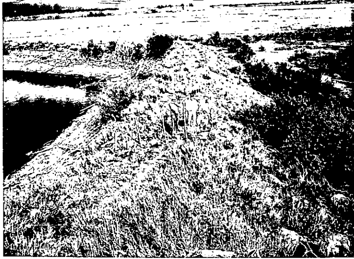
1. Looking northeast along dam axis. Slopes of dam embankment can be clearly seen.
