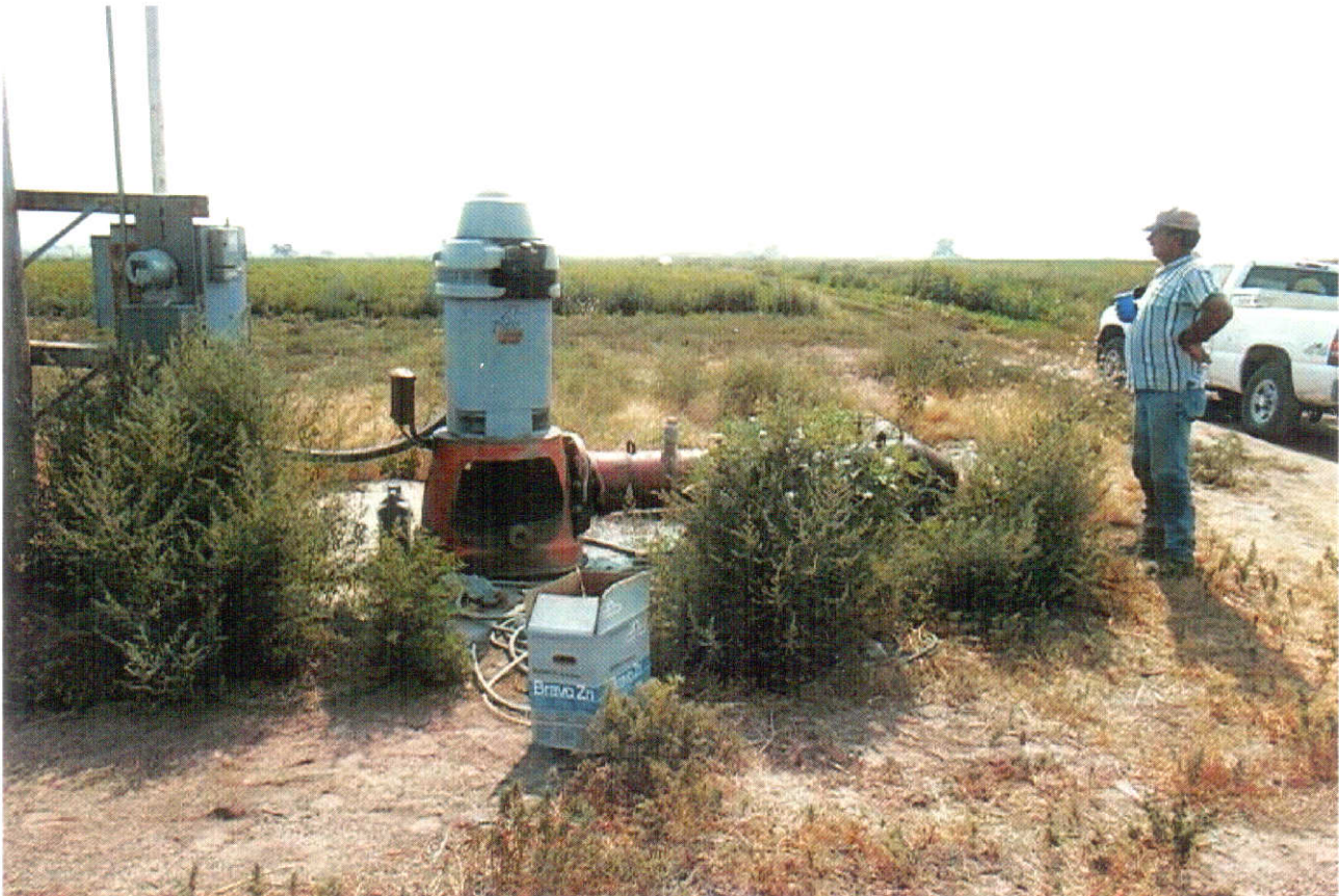
Point of Diversion
