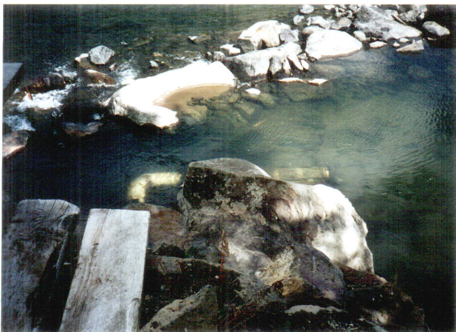
Plate 3 - Inlet pipe and dam from pumping station.
