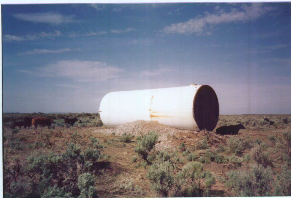
Plate 2 - 10,000 gallon storage tank.
