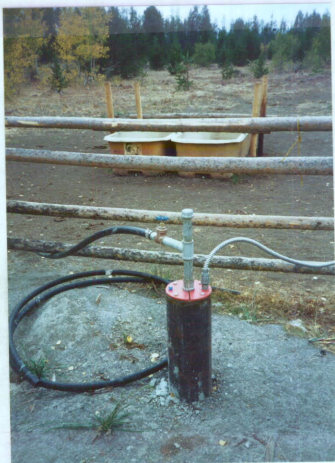
POINT OF DIVERSION FROM INSIDE ENCLOSURE
