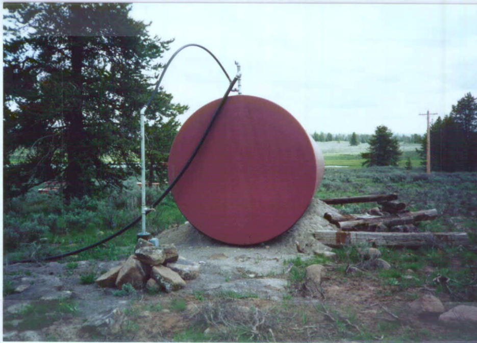
Fig. 1 - Point of diversion with storage tank.
