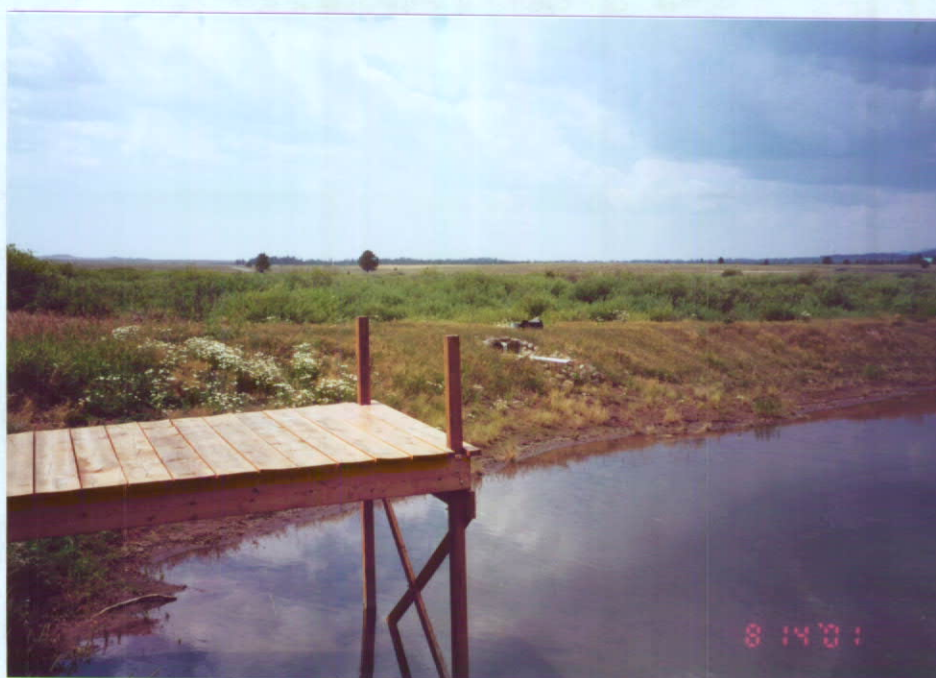
21-7570 - looking at dam (south side of lake)
