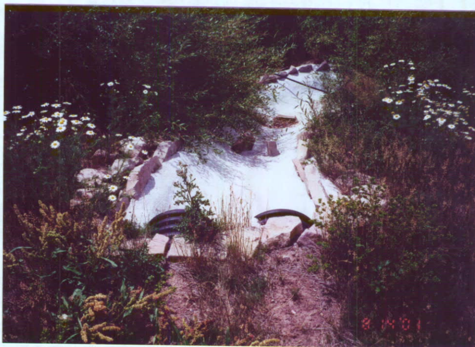
Overflow down to Hotel Creek
