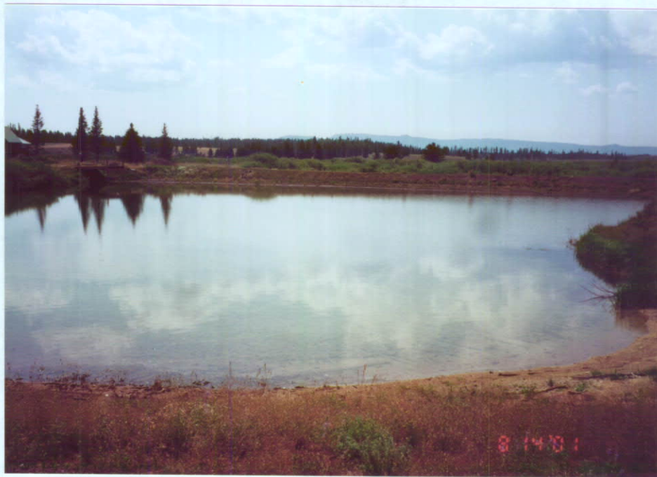
21-7570 POU looking west toward dam.
