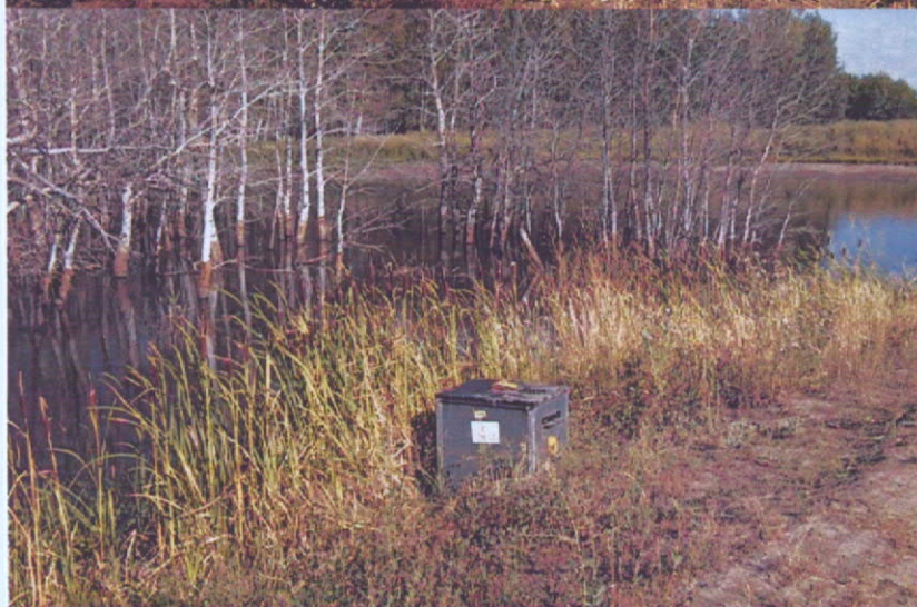
GPS on outflow control box. This box is near center of dam.
