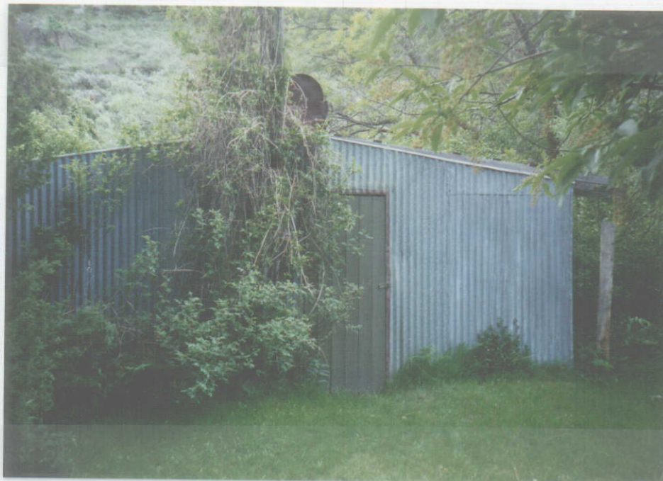
Fig. 2 - Pumphouse along Moody Creek.
