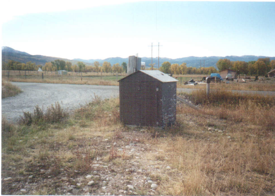
Pumphouse on Robert J. Lyons property.
