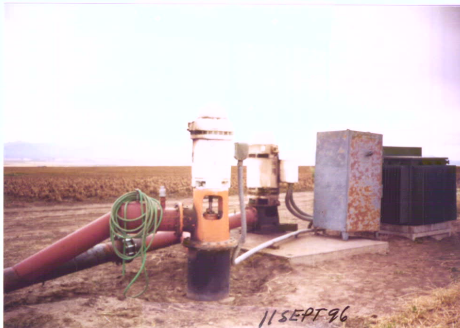
Point of Diversion - Looking East
