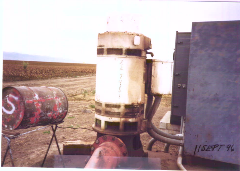
Point of Diversion - Looking Southeast
