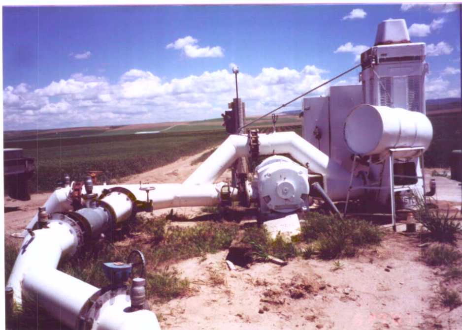
POD # 22-7518 Facing east
