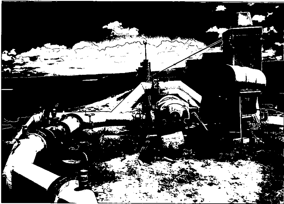
POD # 22-7518 Facing east
