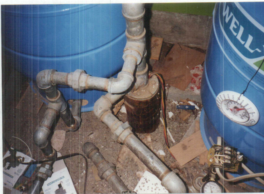
Plate 1 - Point of diversion.
