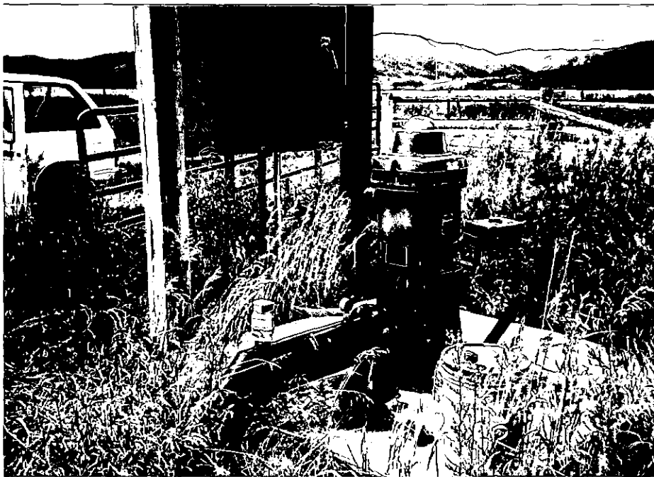
Plate 3 - Motor and pump assembly at point of diversion.
