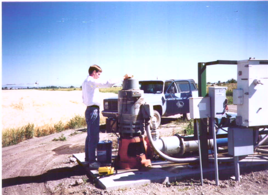
Plate 1 - Point of diversion looking north showing field agent recording GPS location.
