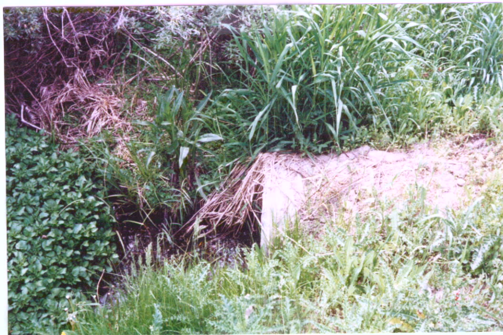
outlet from overflow pipe
