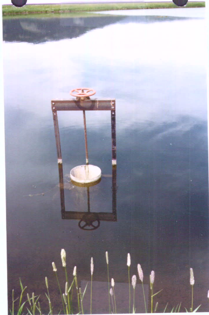
Pond (approx 2 surface acres) with overflow pipe
