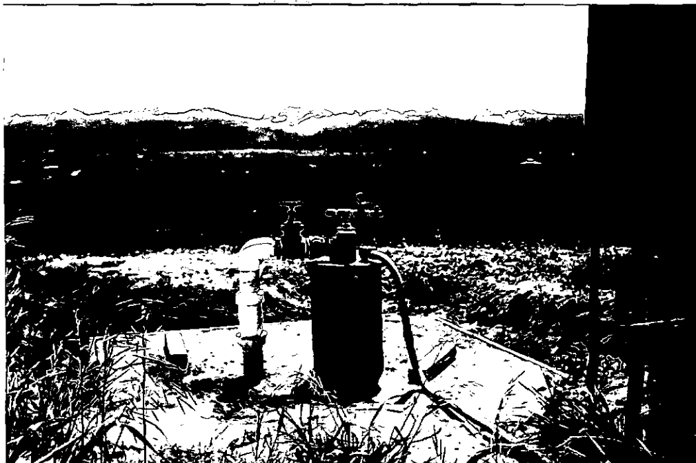
well with 30hp subm. pump, (looking East) 18" casing
