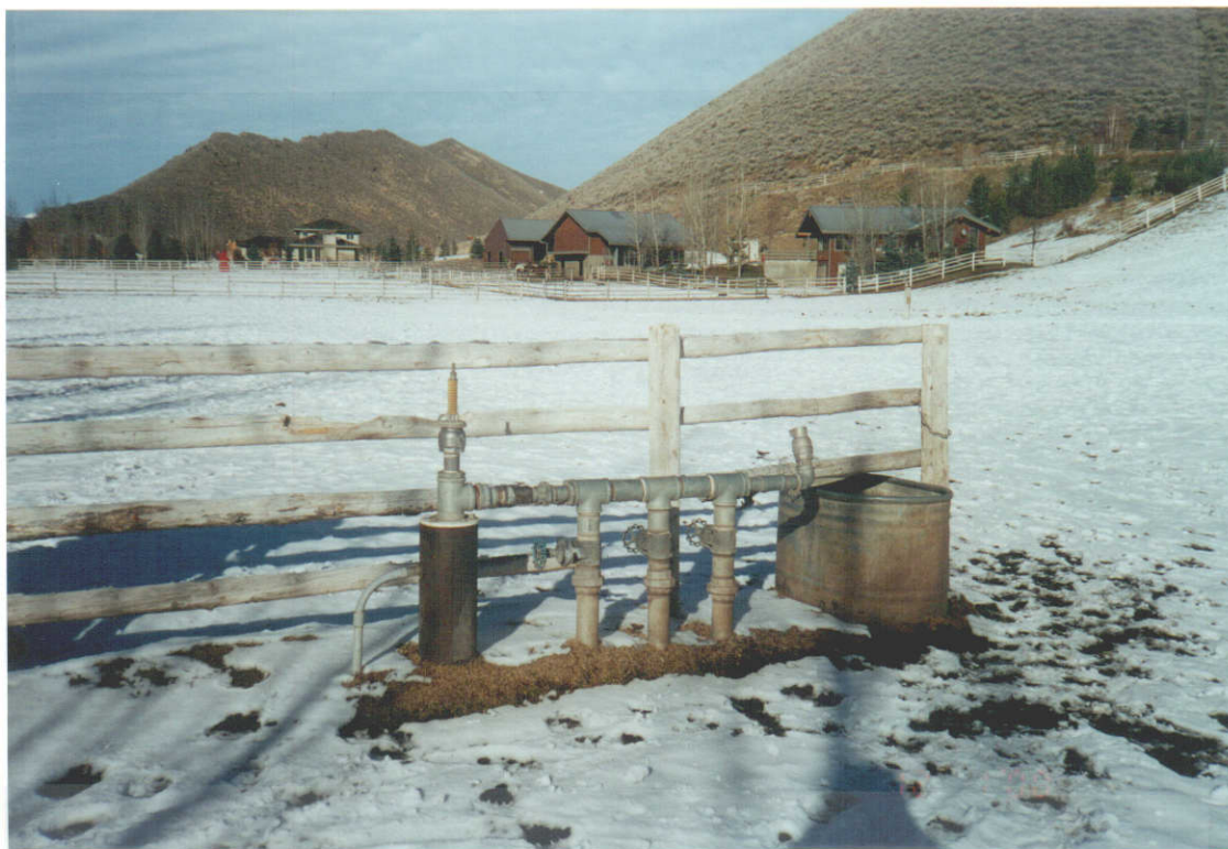
Diversion Works (Looking NE) (Lot 9 Behind Fence)
